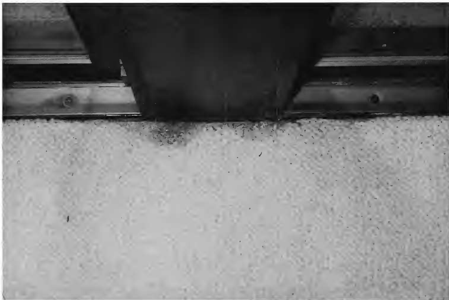
Figure 3. Photograph shows damage caused by plaster bagworm to edge of carpet adjacent to a sliding glass door.
